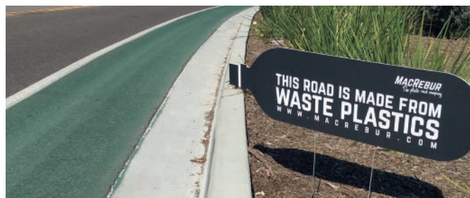
▲ Figure 19.42 Plasphalt is made up of grains of plastic produced from unsorted plastic waste. This replaces the sand and gravel usually used in asphalt production for road surfaces. It can also contain recycled glass pellets
